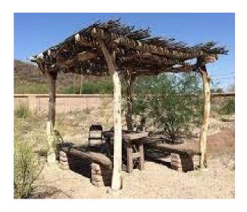
Panels for gates, fences, shade structure roofing are generally wired together using baling wire that can be purchased at any hardware store.
